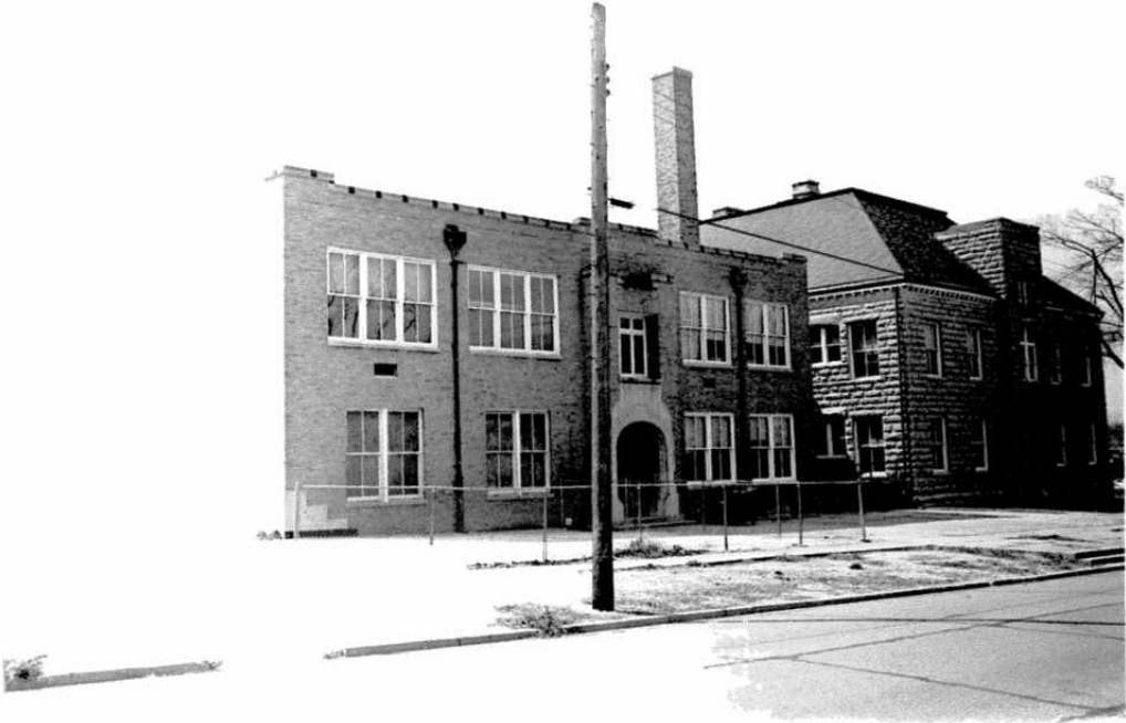
Below: View from northeast of newer building (built in 1927)
